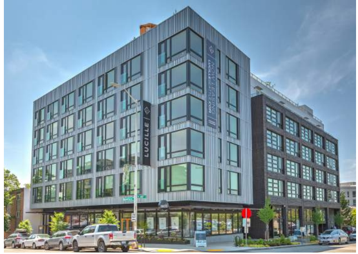
Left). Even with a simple material and color palette, the building utilizes a central massing break to create two symmetrical but smaller building frontage elements to avoid a monolithic frontage. (Right). Building utilizes an asymmetrical break and change in material to provide variation in the facade plane.
