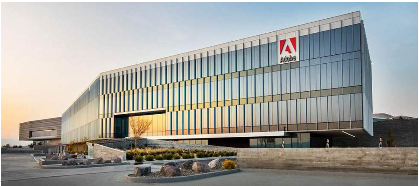
(Top Left) Office design included covered walkways made with perforated metal screens to reduce solar heat gain from the southern exposure. (Top Right). The unique form of the building gives the impression a 'shed' structure floating over a glass box, with vertical circulation (elevator and stair tower) being celebrated with a mural as well as breaking down the horizontal scale of the building. (Bottom) Office building with a flat roof line utilizes vertical fins, cantilevered upper floors, recessed wall areas, and angled facades to create facade articulations and visual interest.
