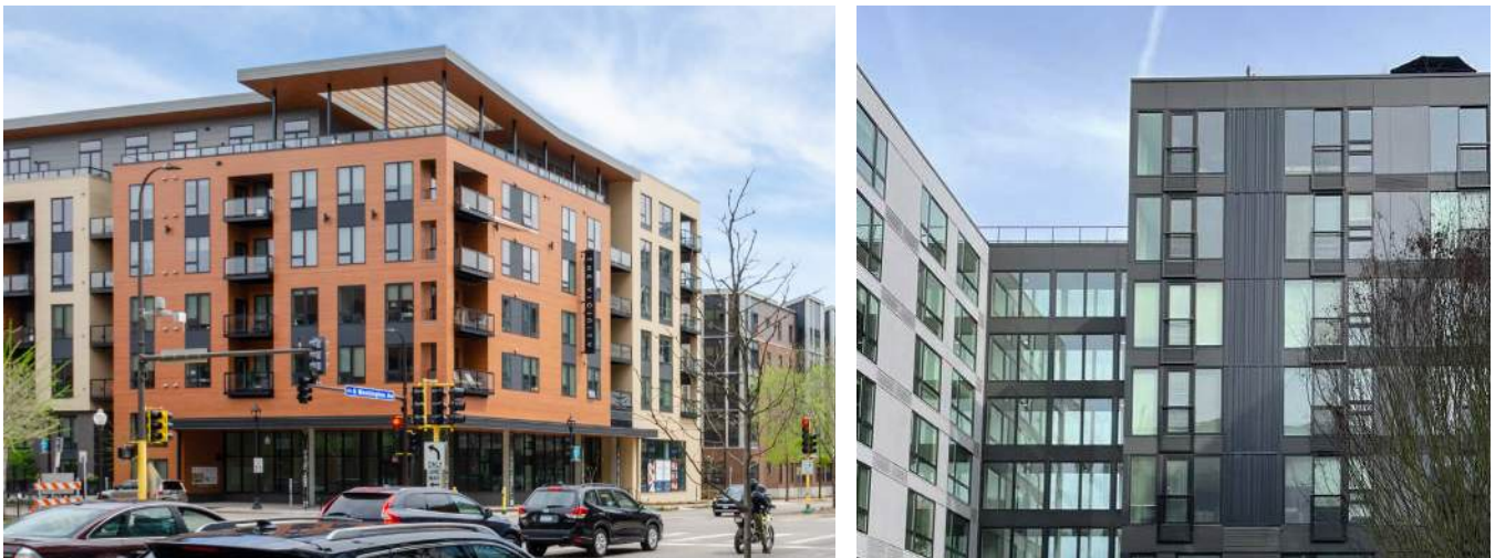
(Left). Building composition includes recessed elements and a step back on the top floor for a corner rooftop amenity covered with a unique canopy structure. These features bring visual interest and enhance the overall public realm experience providing an elevated amenity space with an outward public expression. (Right). The break in the building creates small building massing of differing material compositions while introducing natural light by exposing the corridor and creating visual connections with the external environment.
