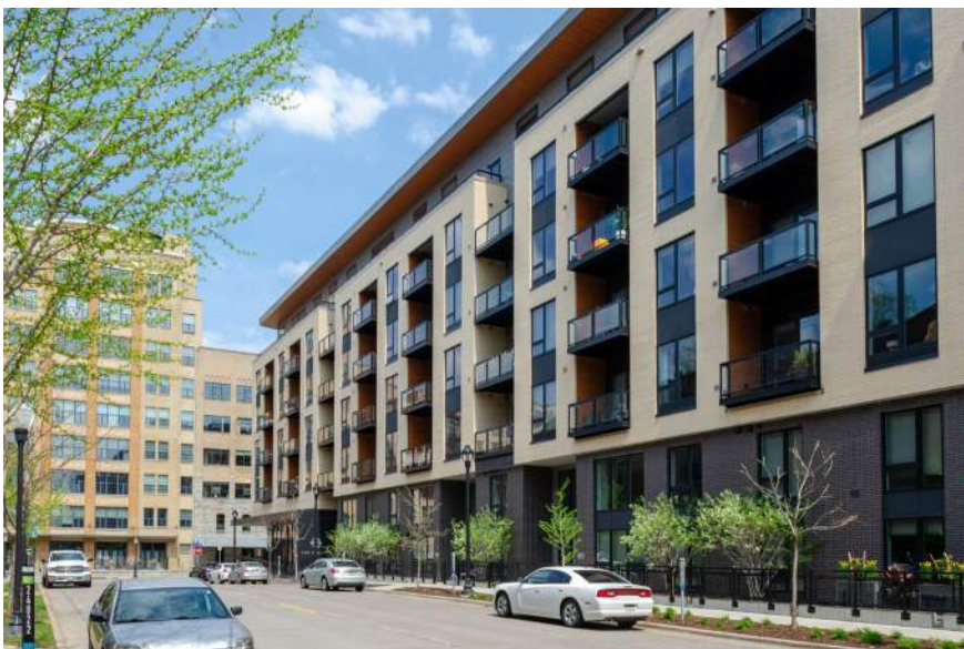
(Left). Recessed balconies are utilized to create unique patterning within the building facade. (Right) Building uses projecting balconies to create depth and articulation within the building facade.
