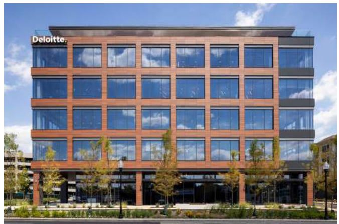
(Left). Glass is used to contrast more solid facade planes, create feature elements compositionally that illuminate differently at night, and to bring focus to primary building entries. (Right). Rooftop step back creates movement in the roofline of the building.
