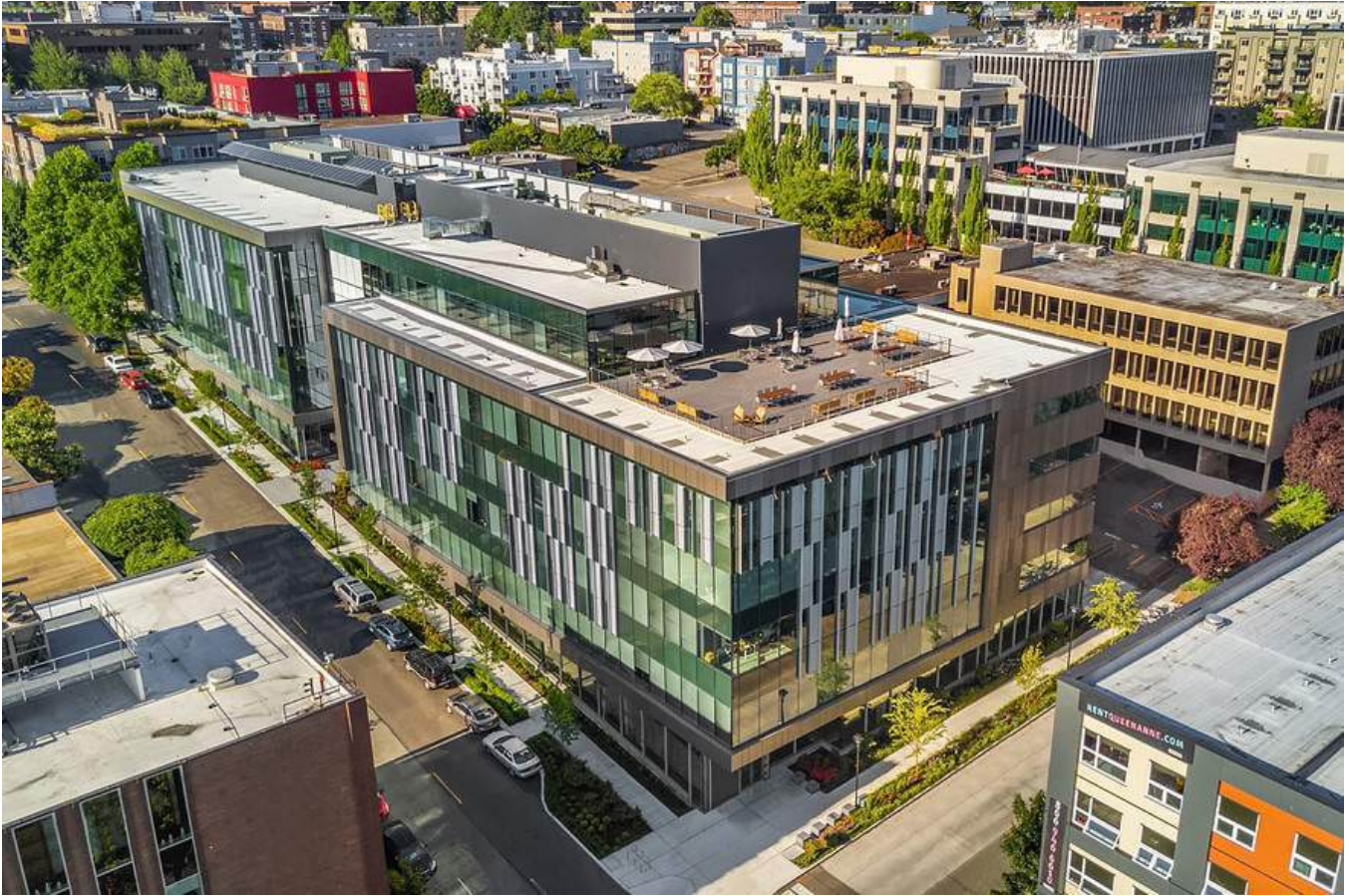
(Above) Mechanical and utility equipment is screened behind tall parapet walls with materials and colors designed to blend into the overall buildings design and composition.
