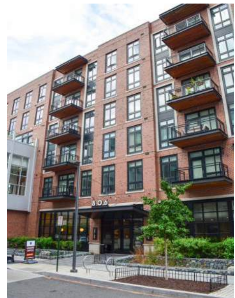
(Left). Recessed balconies are utilized to create unique patterning within the building facade. (Right) Building uses projecting balconies to create depth and articulation within the building facade.
