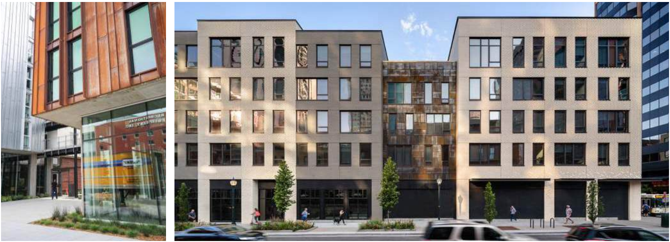
(Left). Recessed base, increased use of glass, and material change helps to distinguish the lower level from the upper floors of the building. (Right). While material changes and how the building expresses itself through the full height of the building to create the impression of a collection of smaller urban buildings, the increased use of glass compared to the smaller window openings on the upper floors of the building help distinguish the base and ground the building.
