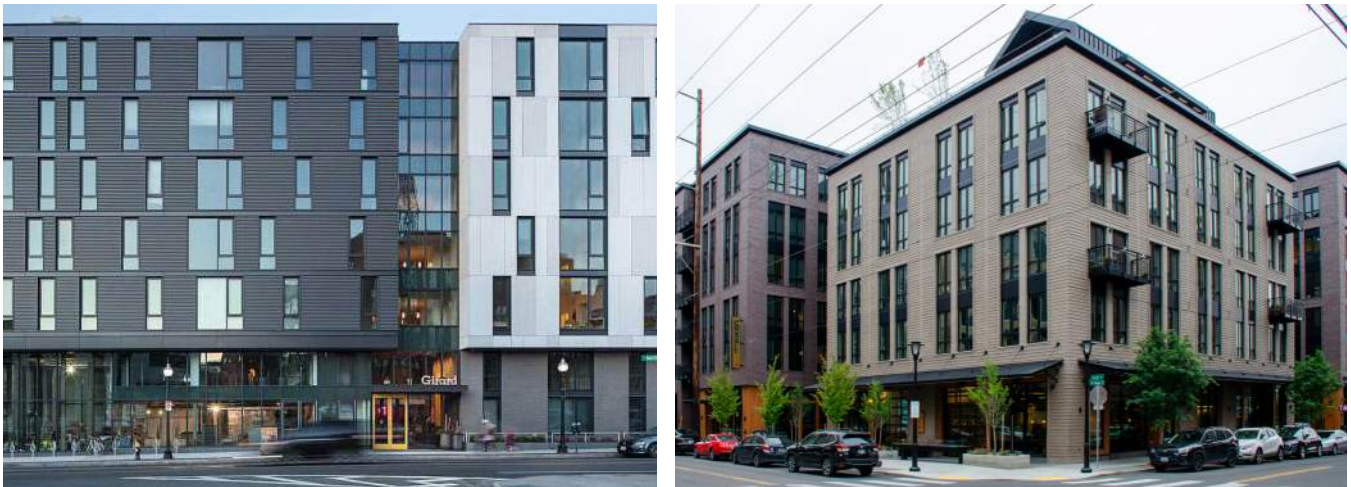
(Left). Building utilizes both a variation in size of windows and staggered window spacing to create visual interest within the facade, while highlighting the resident entrance through more glass vertically expressed. (Right). Building utilizes a more regular grid pattern for windows but groups windows to emphasize vertical expressions in the building facade.
