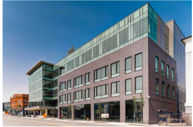
(Left) Office utilizes distinct fenestration patterning on the upper floor, recessed base, and enhanced glazing at the entry that connects to a rooftop amenity to create building articulation. (Right). Building composition includes several changes in facade plane creating movement and depth while emphasizing the corner condition.
