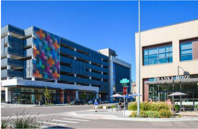
(Left) Example of exposed parking structure in pedestrian-oriented urban neighborhood that utilizes a series of decorative panels, feature walls, and changes in facade plane to create a visually attractive parking structure. (Right). Parking structure facade is organized compositionally like a building with a distinct base, fenestrations, and a series of feature walls of varying materials, one of which was used for signage.
