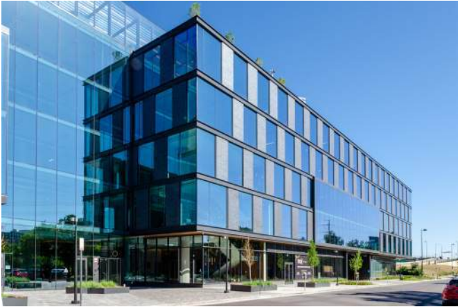
(Left) Office utilizes distinct fenestration patterning on the upper floor, recessed base, and enhanced glazing at the entry that connects to a rooftop amenity to create building articulation. (Right). Building composition includes several changes in facade plane creating movement and depth while emphasizing the corner condition.
