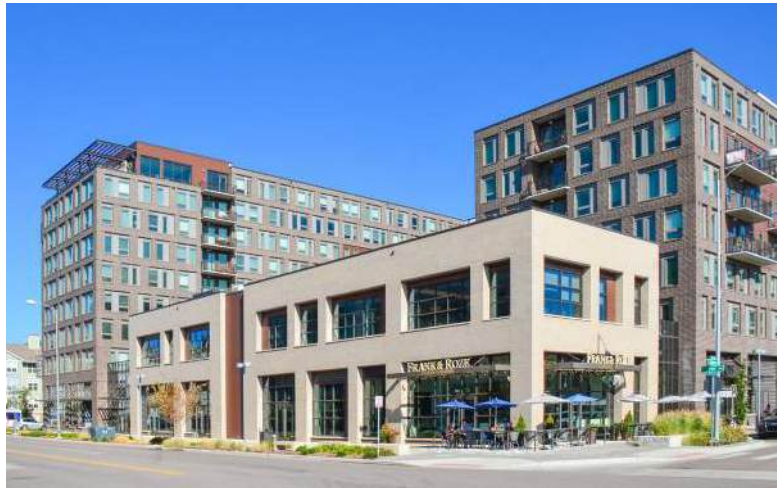
(Left). Sawtooth treatment of the roofline gives a distinct form to the building. (Right). Building design uses smaller building forms, step downs, and low-rise building forms to create visual interest and movement in the collective roofline of the building.
