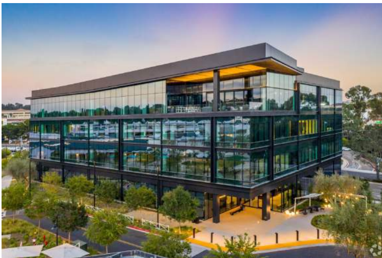
(Left) Darker material palette consists of architectural grade metal panel and glass with two recessed elements, one to highlight the lobby entrance and the other to highlight a rooftop deck. (Right). Lighter material palette consisting of brick, wood metal, and regular window pattern. A building recess provides a common outdoor balcony on each floor, breaking up the buildings massing to create smaller facade elements and creates movement in the roofline.
