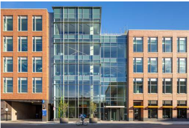
(Left). Glass is used to contrast more solid facade planes, create feature elements compositionally that illuminate differently at night, and to bring focus to primary building entries. (Right). Rooftop step back creates movement in the roofline of the building.
