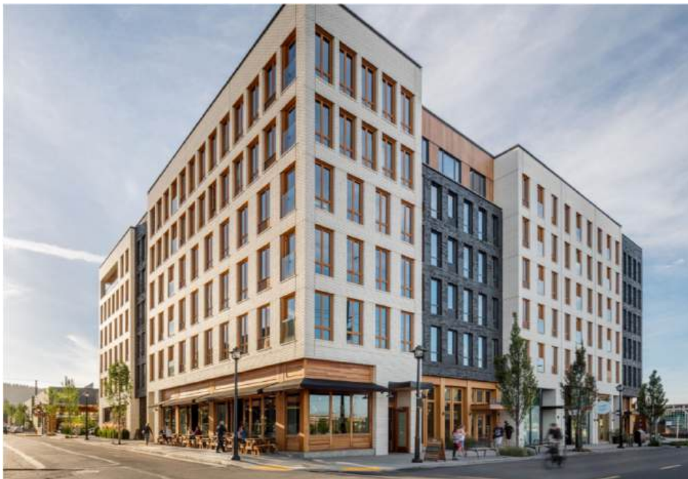
Figure 3. The apartment building includes a flat roof design with varying parapet heights and an architectural hierarchy to the street corner.
