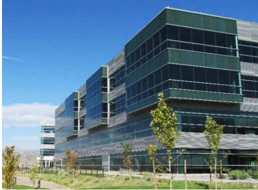
Figure 126 – The metal used on this building is of a high grade and provides an architectural quality to the building.
