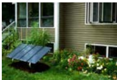
Ground-mounted solar array allows optimal tilt and avoids placement of panels over roofing.
