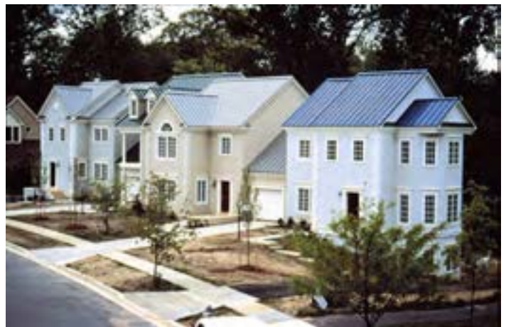
Flexible thin film solar panels blend in between the ridges of metal roofing.
