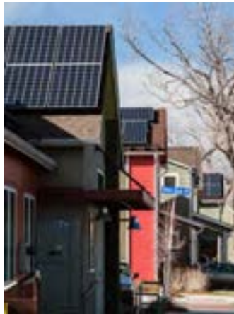
Shading can greatly affect power output. Examine effects of seasonal sun angles, new buildings and growing trees.
