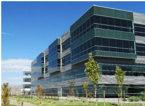
Figure 84 – Metal used is of a high grade and provides an architectural quality to the building.
