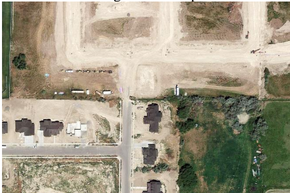
Figure 154. Subdivision under construction is connecting to an existing street stub.
