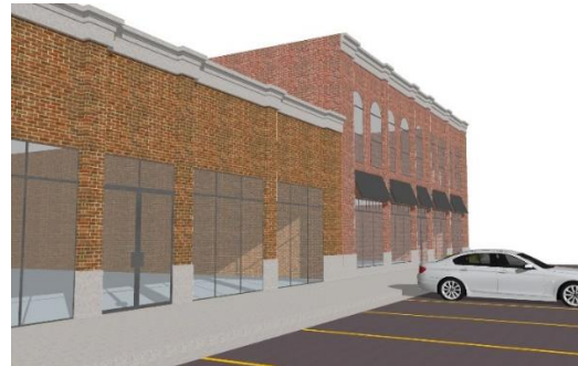
Figure 21 – Inappropriate lack of landscaping leaves the rear side of the building with only impervious and hard surfaces.
