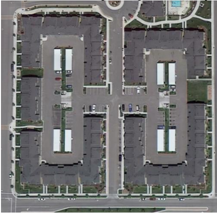
Figure 139. Apartment development with parking located on the interior portion of the site with buildings oriented to the streets.
