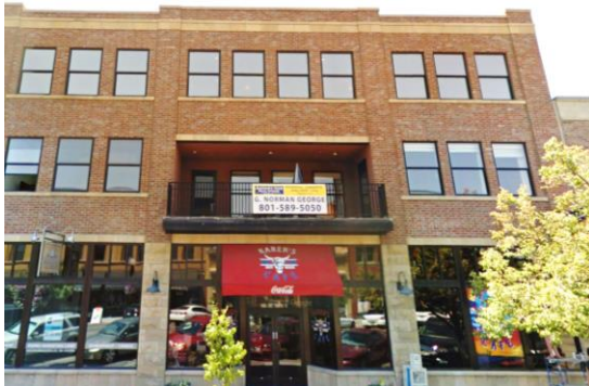
Figure 4. Building rooflines are flat with parapet extensions to create a varied roofline.
