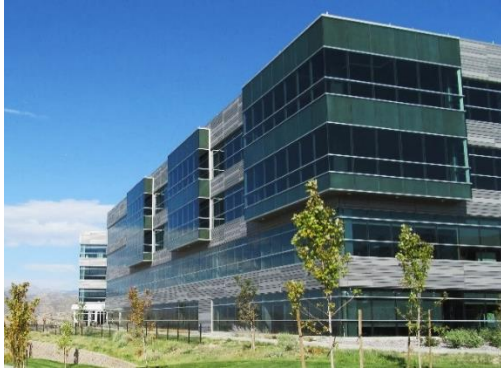
Figure 66 – Metal used is of a high grade and provides an architectural quality to the building.
