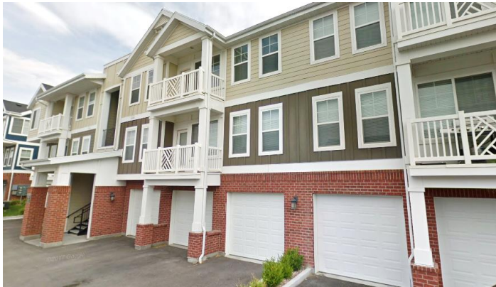
Figure 15. Tuck-under garages are built into the rear side of the principal structure to provide off-street parking while limiting the amount of surface parking areas.
