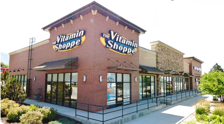
Figure 37. Stucco is only applied to recessed and secondary wall areas, and the hierarchal features use brick and rock.
