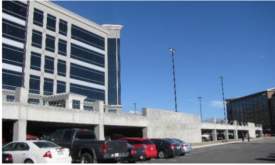
Figure 175. The parking structure facade exhibits variations with the use of embossed concrete walls and the use of pillars and cable.
