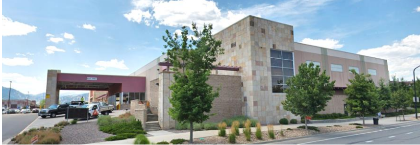
Figure 76. The street side of this regional retail building includes glass used as an accent. The façade also utilizes articulation in the facade and roofline, changes in material, and canopies to provide architectural interest that addresses the street.
