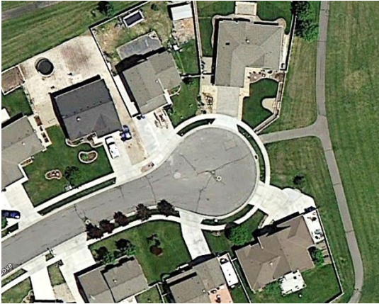
Figure 150. Cul-de-sac with a pedestrian connection to allow access to an adjacent open space.
