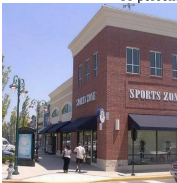
Figure 62. The first floor facing the street includes large clear glass windows.
