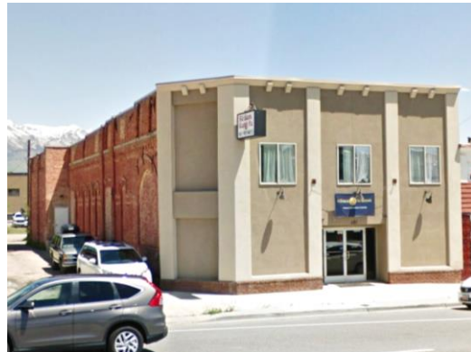
Figure 25 – Existing building with inappropriate updating and remodeling that is not consistent with the original historic design. Original materials and architectural elements have been covered with a stucco facade.
