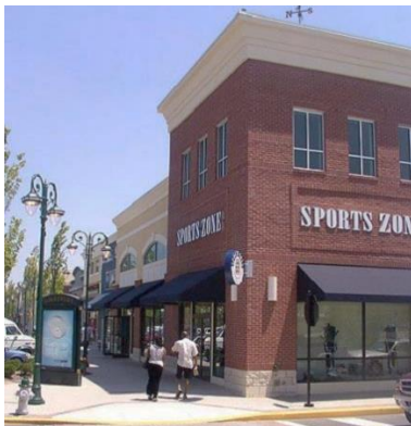
Figure 44. The first floor facing the street includes large clear glass windows.
