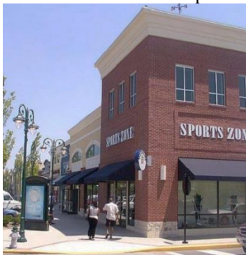
Figure 75. The first floor facing the street includes large clear glass windows.
