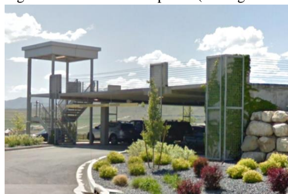
Figure 178 – The parking structure support columns use trellis features for vines and greenery to grow vertically.
