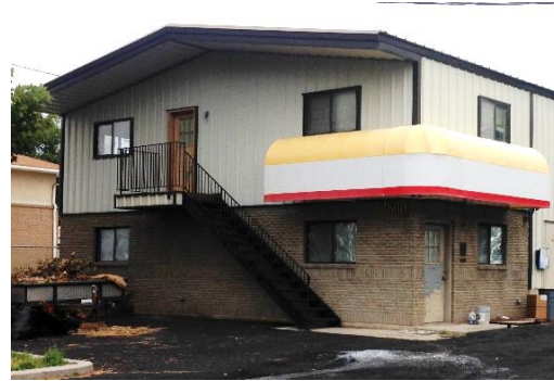
Figure 54 – Metal used is an industrial grade and has the appearance of standing seam metal which detracts from the architectural quality of the building.
