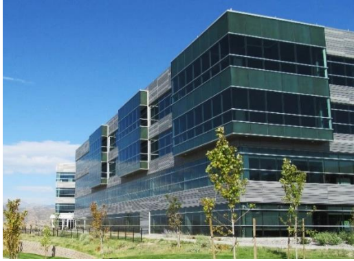
Figure 126 – The metal used on this building is of a high grade and provides an architectural quality to the building.
