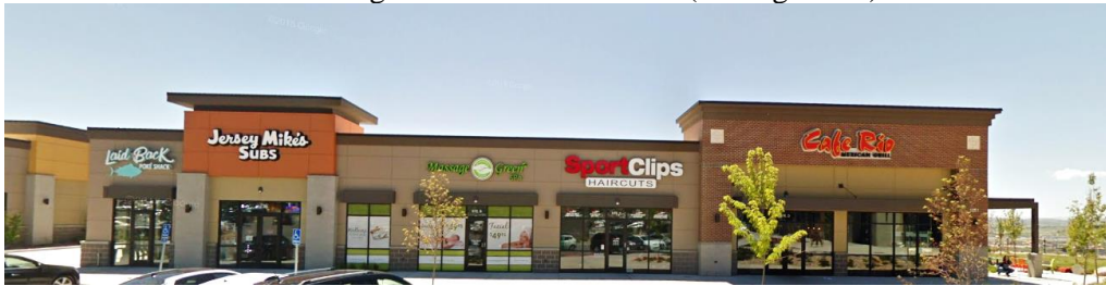
Figure 45. Two hierarchal building features are included on this building for separate entrances.
