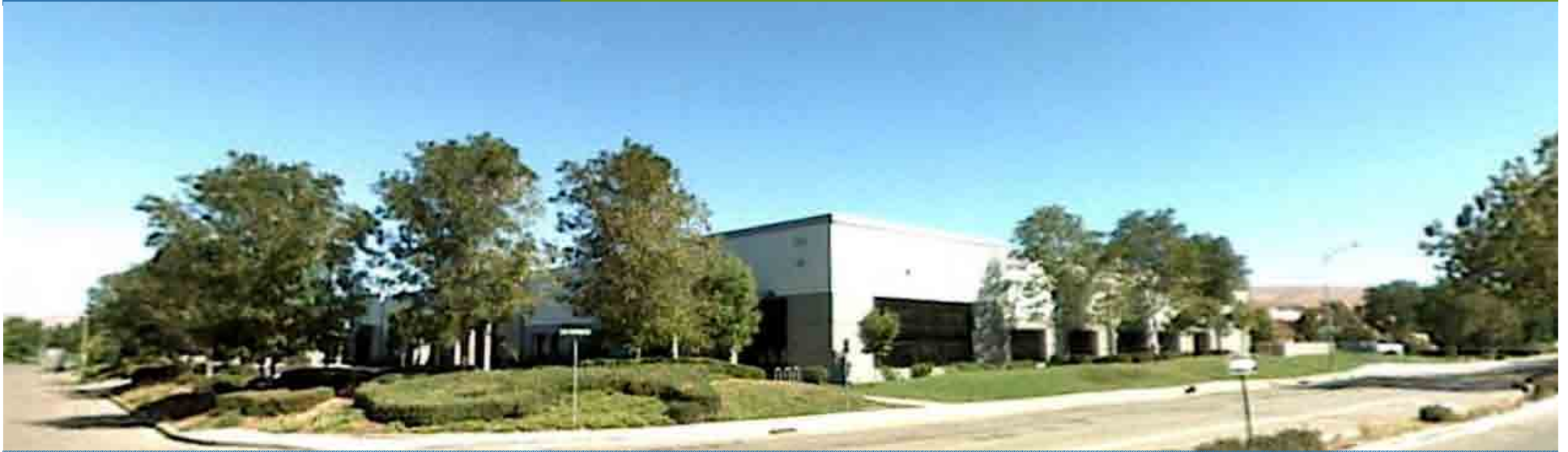
Fig. 1. Light industrial sites to have wide, generously landscaped setbacks, as well as pedestrian sidewalks.
