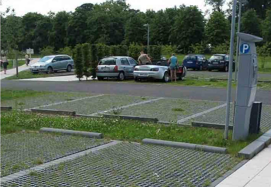
Fig. 1. Pavement should be highly reflective and, where possible, pervious.
