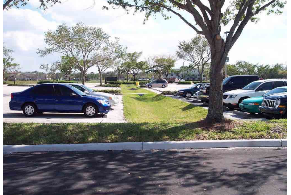
Fig. 2. Swales help manage stormwater runoff.
