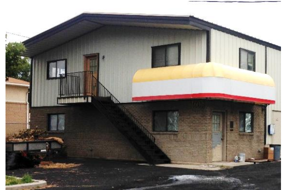
Figure 127 – Metal used is an industrial grade and has the appearance of standing seam metal which detracts from the architectural quality of the building.
